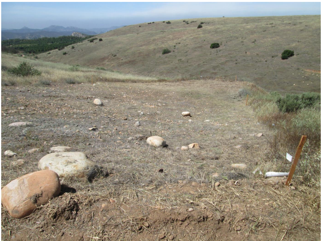
Photo 5: Stringing site (pictured) and helicopter landing zone work limits were delineated with wooden stakes in accordance with APM BIO-1 and vegetation trimming occurred only within the delineated work limits.
